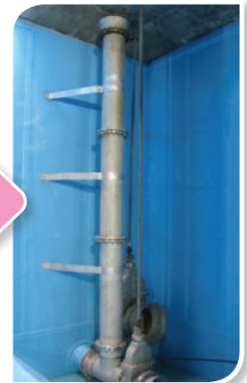
After installing collecting well
