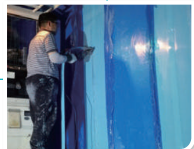
Fusion of the Connecting Area of Panels
