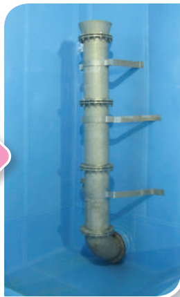
After installing collecting well
