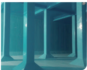
Completion (SPEP panel lining reservoir)
